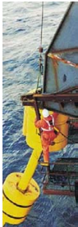
Flexible-joint connecting the first SCR (steel catenary riser) designed and installed in Brazil, to the semi-submersible platform Petrobras18.
